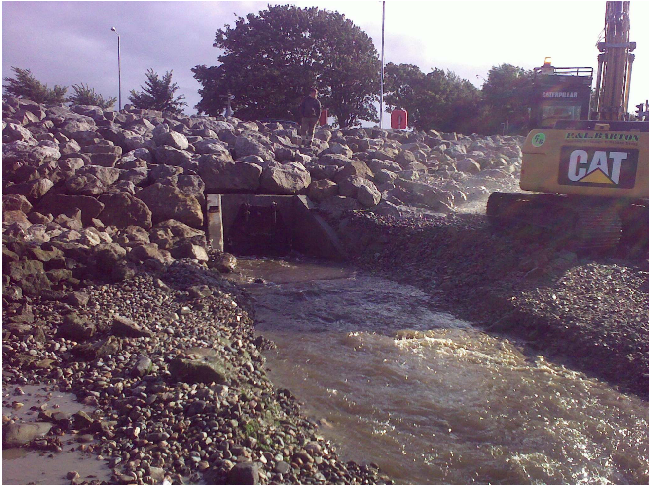
Bare Beck outfall after clearance.
